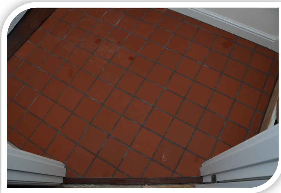
Figure 8 - Floor laid with unglazed quarry tiles
